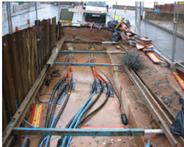
Figure 1.3 Typical Onshore Underground Cable Connection Pit
