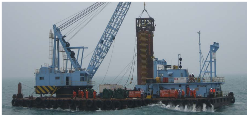
Figure 1.9 Suction Caisson Test
